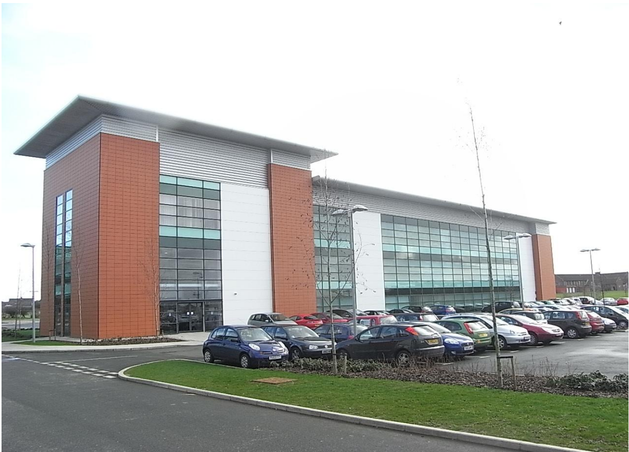
The Q16 Building, Quorum Business Park, Newcastle
